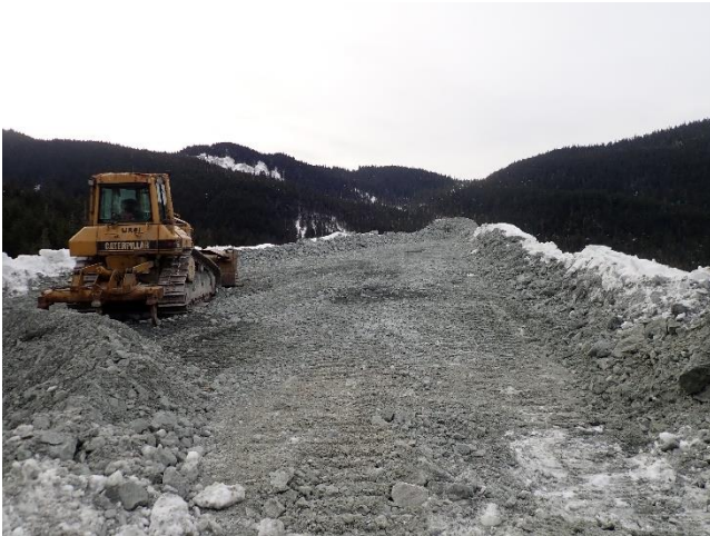
Photo 2. The Comet development pile.
