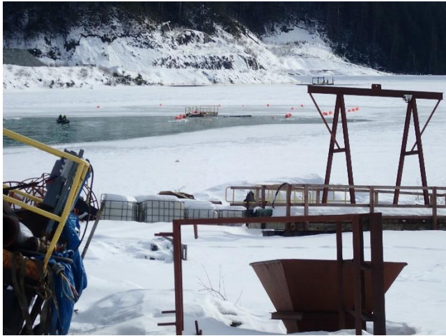
Photo 17. TTF personnel were in the process of breaking ice.
