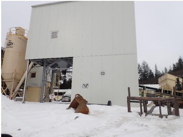
Photo 14. The Pug plant at Pit 4.
