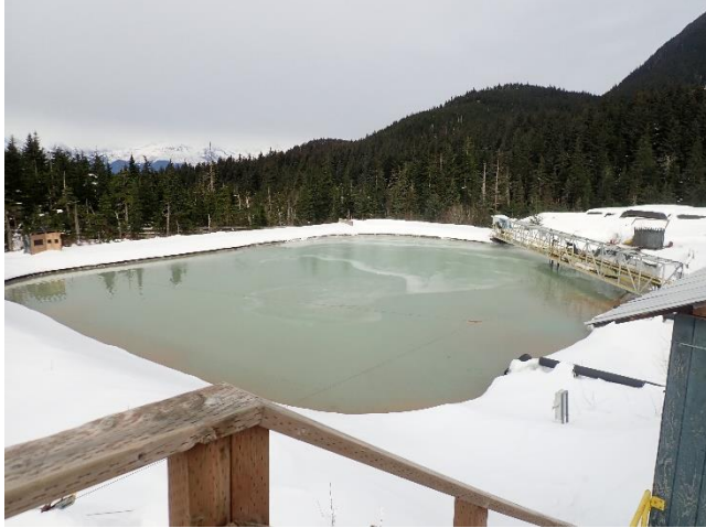
Photo 4. The CWTP's Pond-2.
