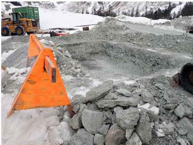
Photo 12. The location for the new refueling pad.
