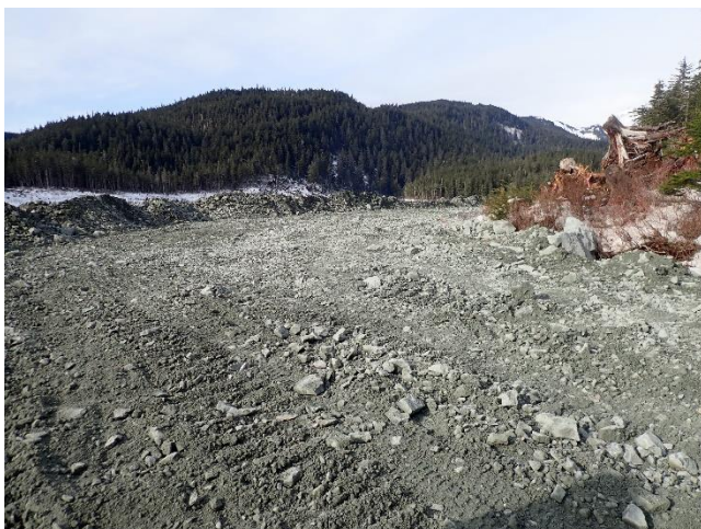
Photo 15. The new TTF access road.
