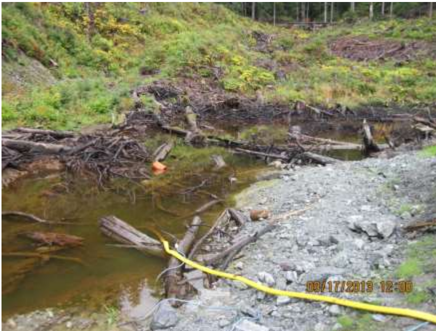
Photo 08. The pH at the northwest pond was about 5.5. Water is being pumped from the pond to the ARD containment pond.
