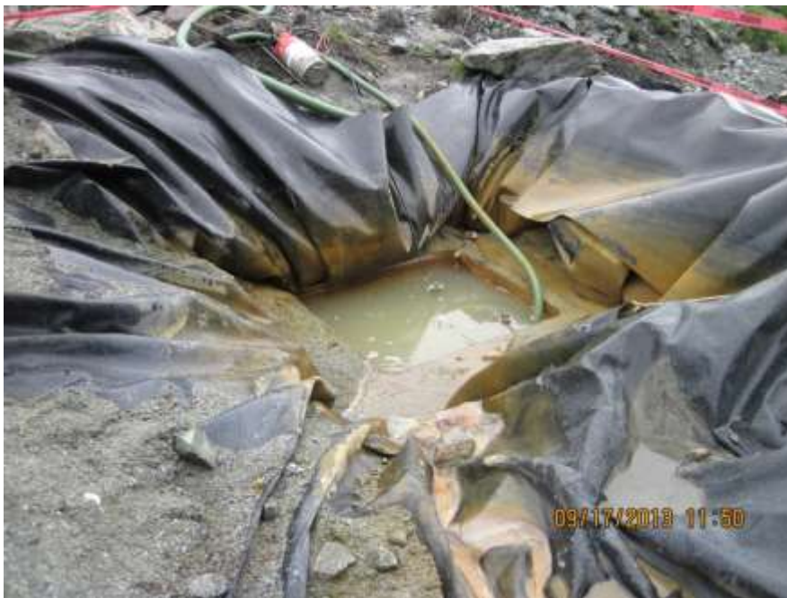
Photo 06. The pH at the sump was about 5. Water in the sump is being pumped to an ARD containment pond, and then sent to the GP water treatment plant.
