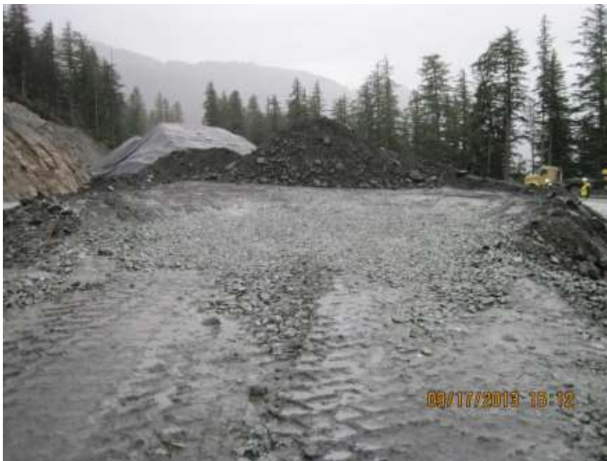
Photo 10. The GP from the cell in the foreground is being hauled underground. The two cells in the background are covered, but not sealed.
