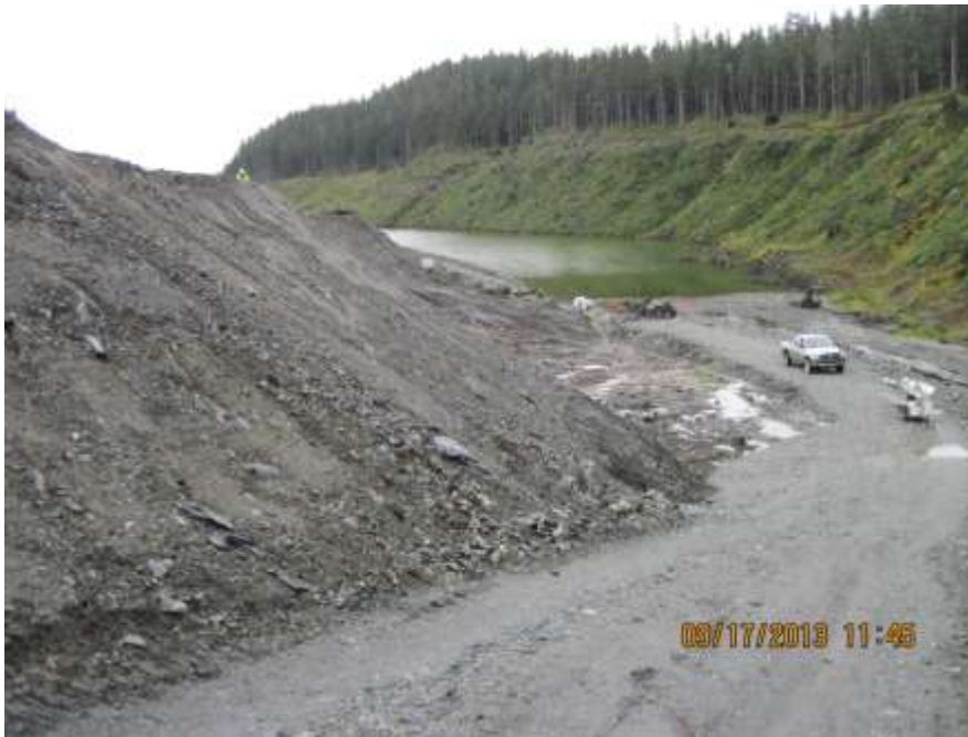
Photo 03. About 14,000 tons of graphitic phyllite have been excavated from the north end of the TTF this summer. Lower Slate Lake is in the background.
