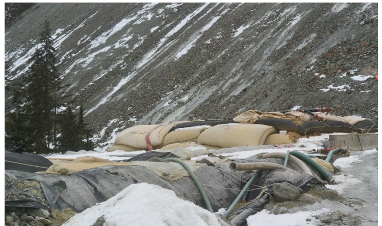
Figure 4 Dewatering bags filled with sediment dredged from the ponds.
