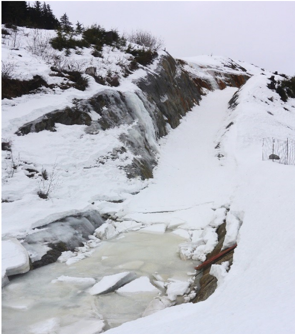
Figure 7 Emergency spillway and plunge pool.
