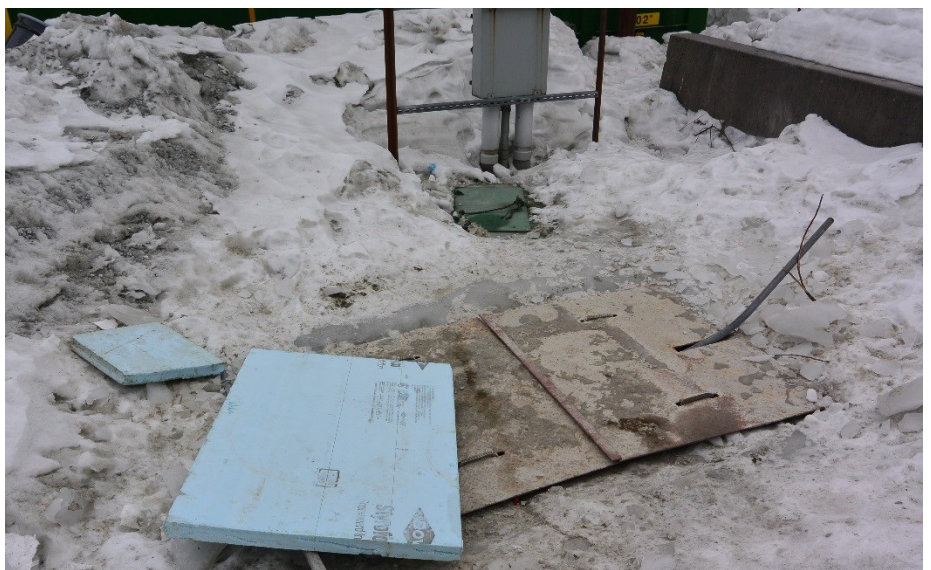
Figure 6 Secondary containment sump and lift station.
