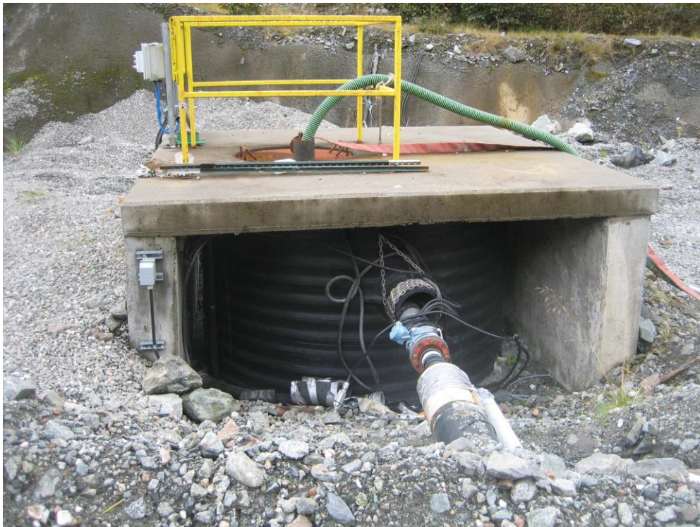
Photo Z Lower Slate Lake Dam Seepage Collection Sump.
