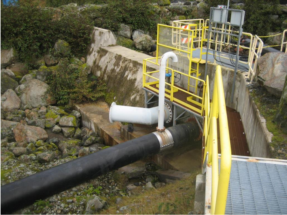
Photo C Upper Slate Creek Diversion Dam
