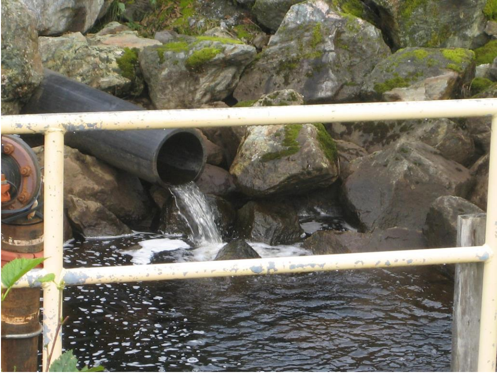
Photo D Upper Slate Creek Diversion Dam
