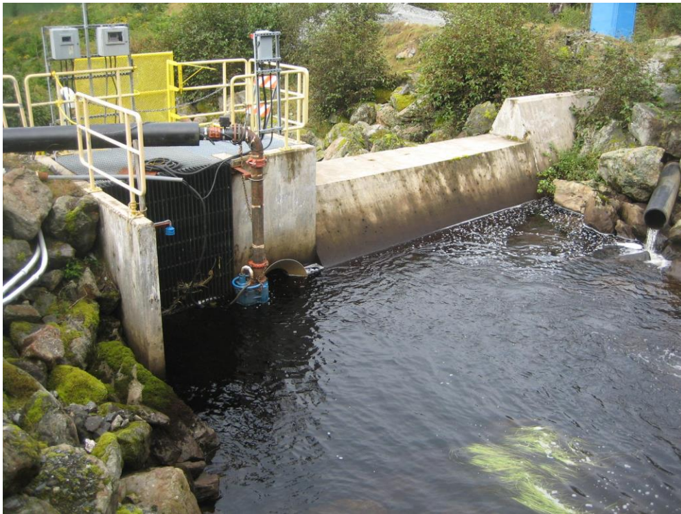
Photo B Upper Slate Creek Diversion Dam
