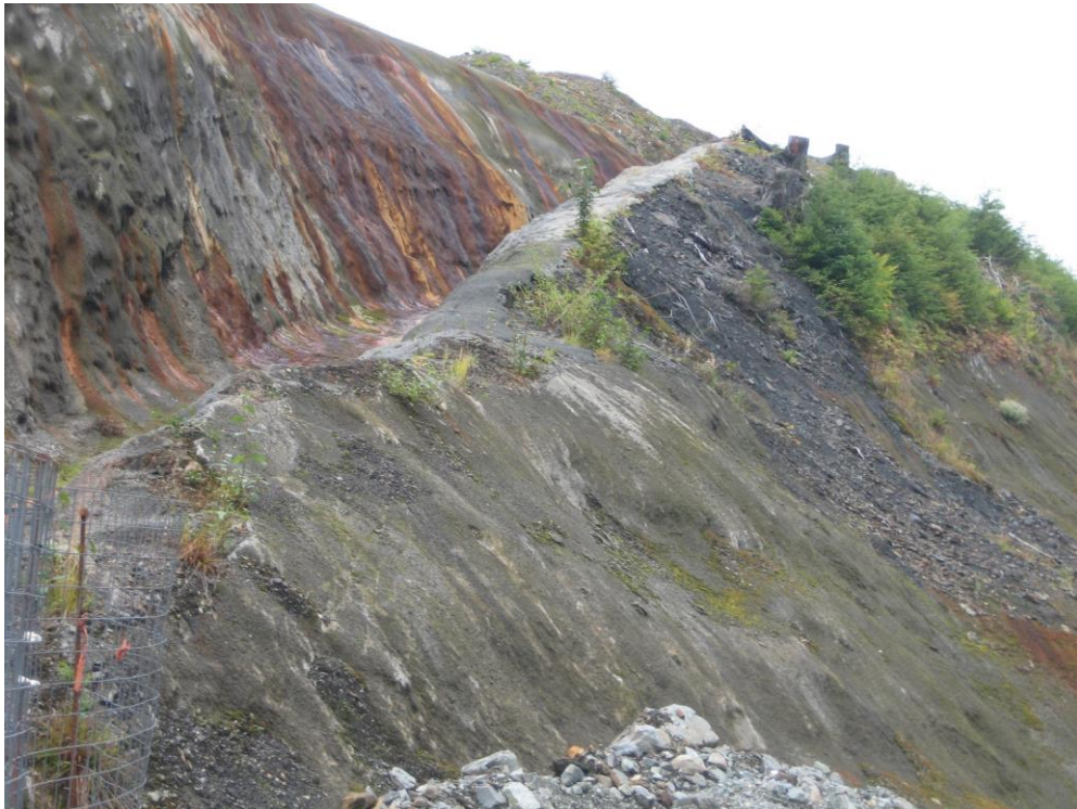
Photo FF Lower Slate Lake Dam collection channel and sump along and downstream of west groin of dam below shotcreted west abutment wall.
