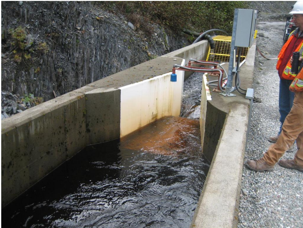
Photo N Parshall Flume for combined flow from Lower Slate Creek Diversion Dam & North Diversions at east (left) abutment of dam.
