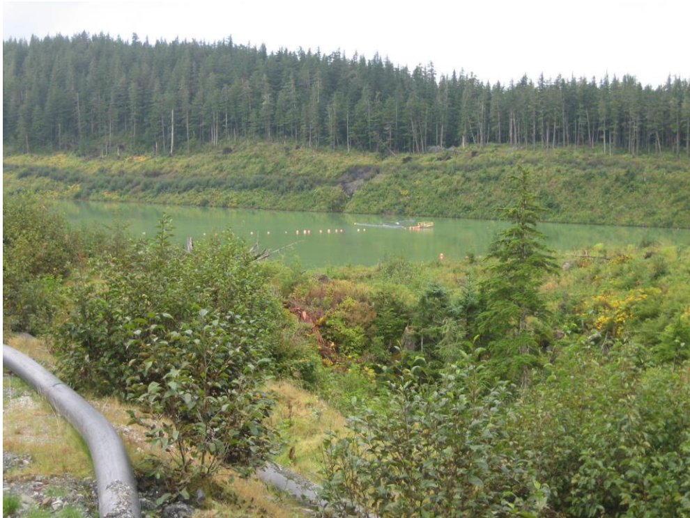
Photo H Lower Slate Lake Tailings Impoundment
