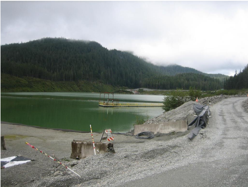
Photo V Lower Slate Lake Dam and Tailings Impoundment, looking upstream (north-northwest).
