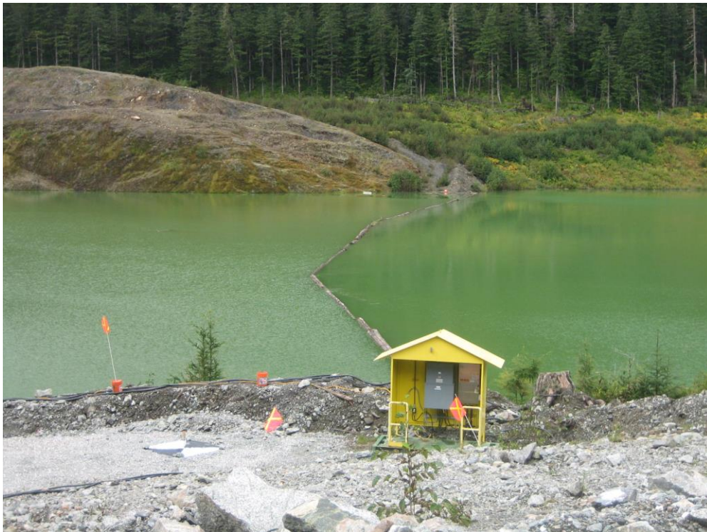
Photo J Lower Slate Lake Reclaim Water Line & Barge pump control shed, cabled log debris barrier behind
