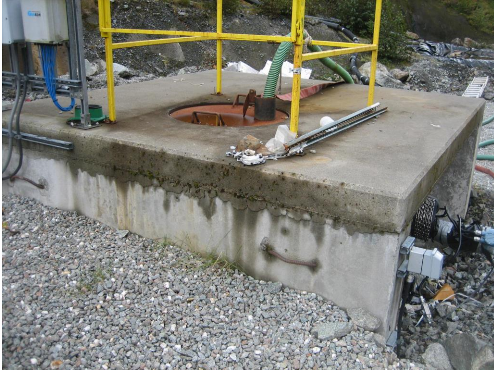
Photo Y Lower Slate Lake Dam Seepage Collection Sump.
