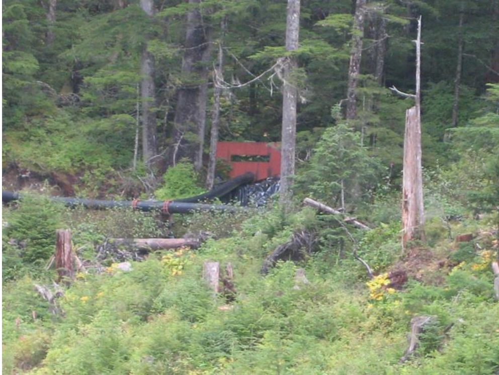
Photo A North Diversion Structure north of Lower Slate Lake impoundment
