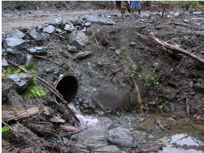
Culvert along road to quarry
