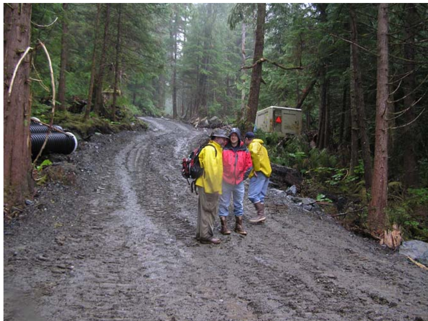
Road from new barge landing
