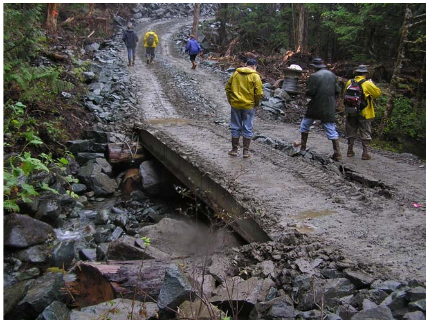
Bridge across Camp Creek
