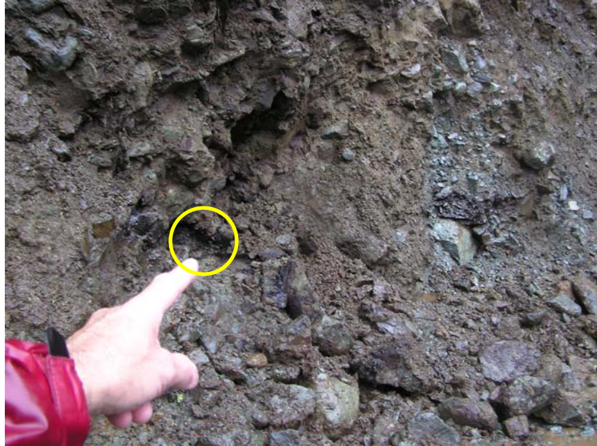
Seep in a "conduit" through the colluvium
