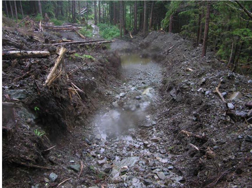
Trench between quarry and area of proposed AG rock storage pile
