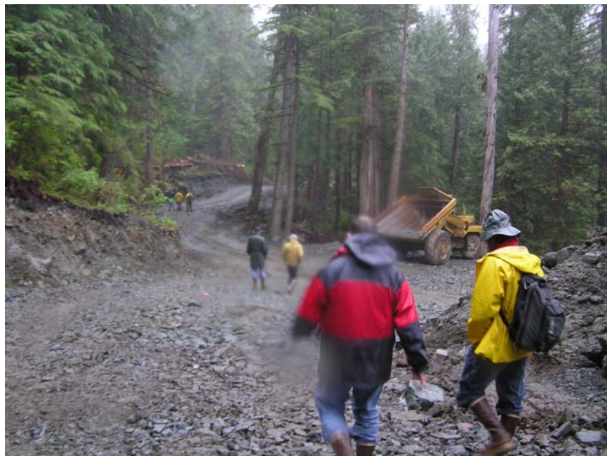
Road to quarry, magazine, and AG rock storage
