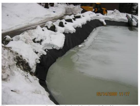
Water treatment system sedimentation basin – inlet pipe at left (~ 20 gpm)
