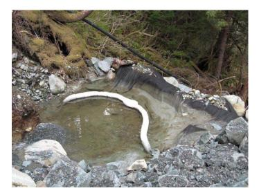
Storm water sediment pond with oil collection boom to capture residual hydraulic fluid from a spill at the mine portal.
