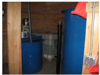
Water treatment plant with lime mixing tank, lime contact tank and flocculant tank.
