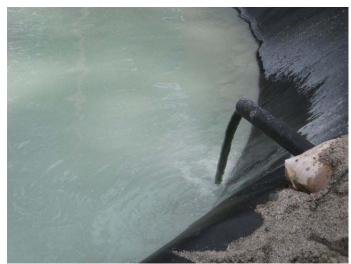
Mine dewatering water entering the first water treatment pond.
