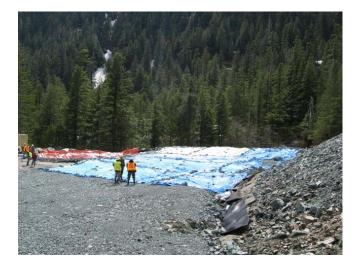
PAG site with PAG waste covered with a blue tarp to shed rainwater. Some seeps through, so future rock will be laid with a surface slope to shed the water.
