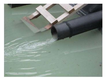
Water partially treated – sediments reduced by the use of flocculants – this water is passing from the first to second treatment ponds.
