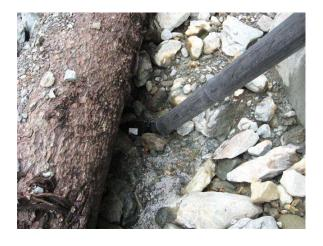
Repaired joint of mine dewatering pipeline – this joint came apart in January 2008.
