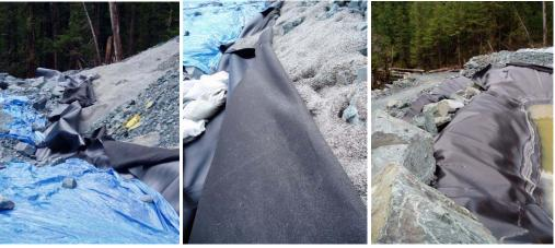
Liner system showing sand, geotextile and geomembrane. Right photo shows how the liner is anchored.
