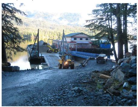
Photo 14. Barge ramp, float dock, and floating barge camp.
