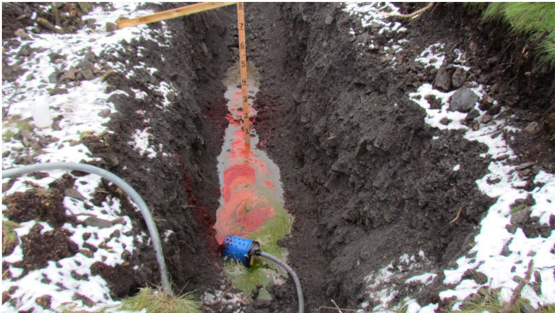
Figure 9. Eosine dye introduction into Trench T-3.
