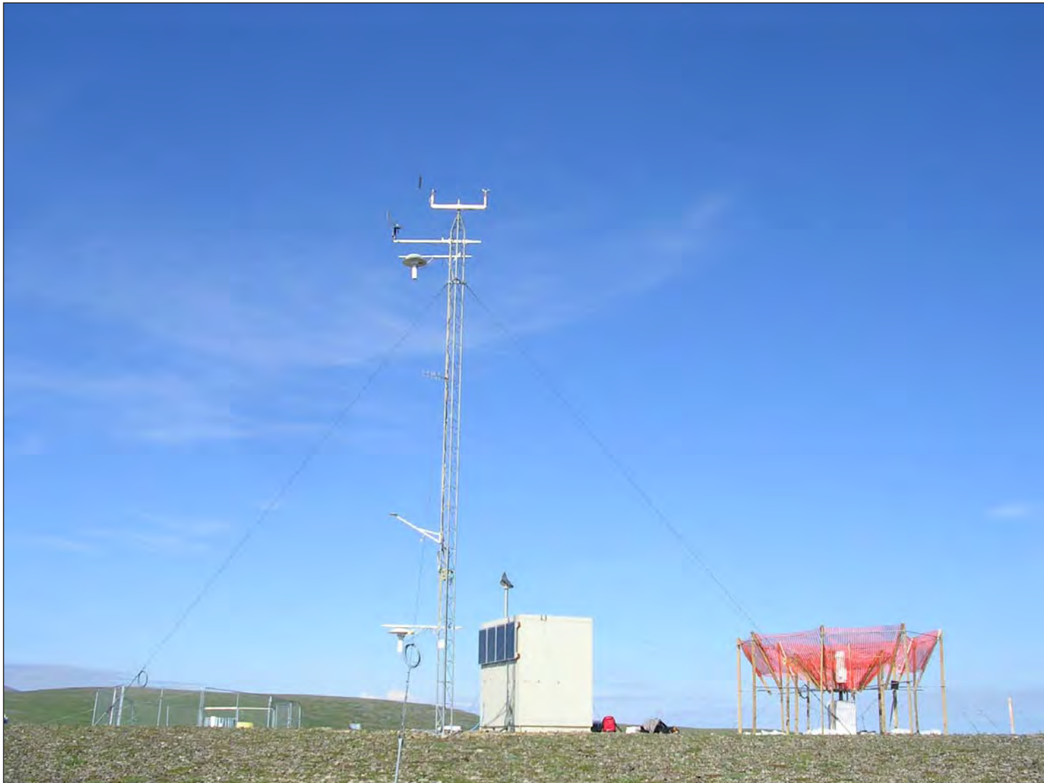
Figure 1-3. Pebble 1 Meteorological Monitoring Station.
