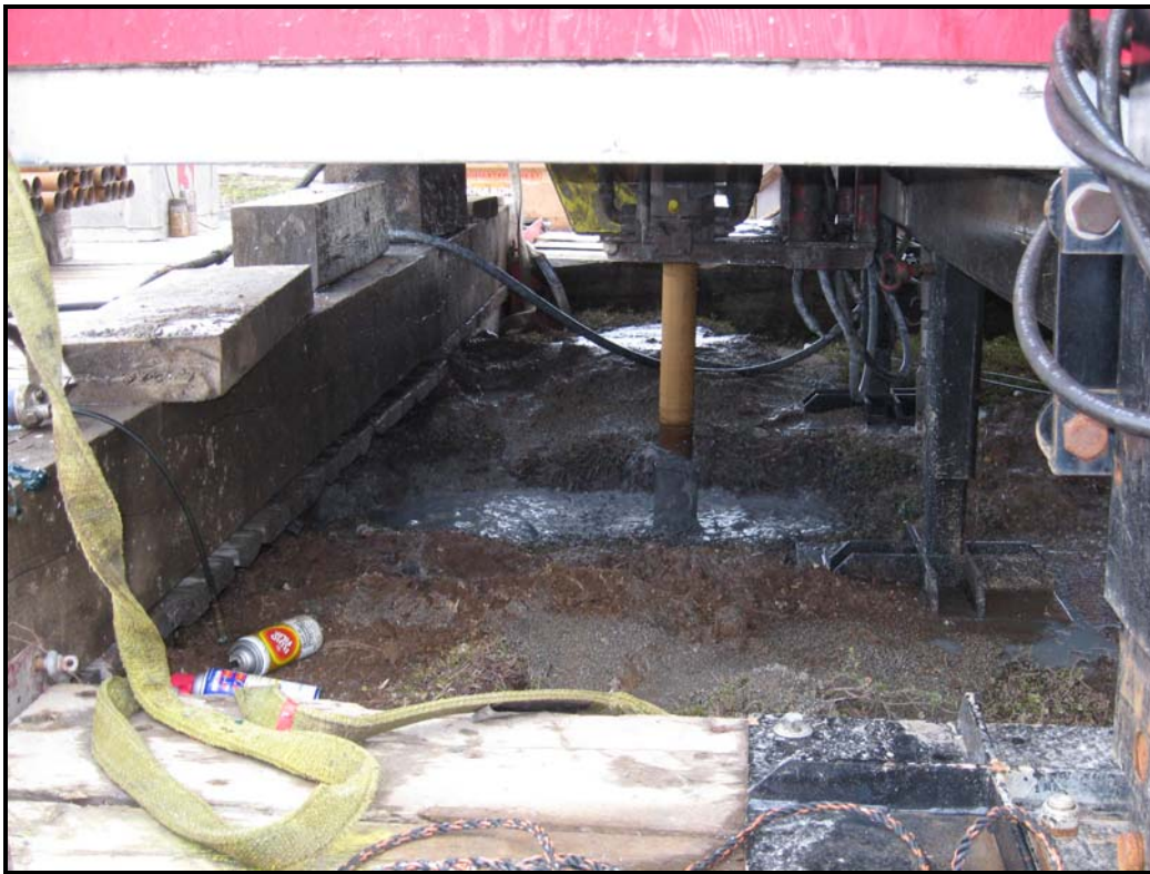
Figure 2. Active drill currently at a depth of 928 feet, going to 1200 feet.
