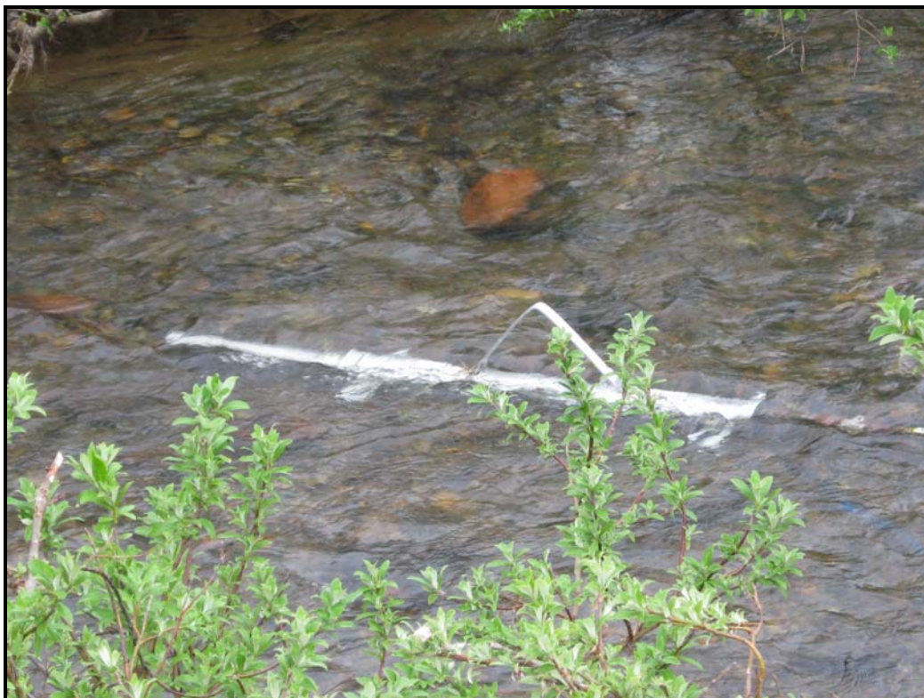
Figure 8. Screened water intake structure.
