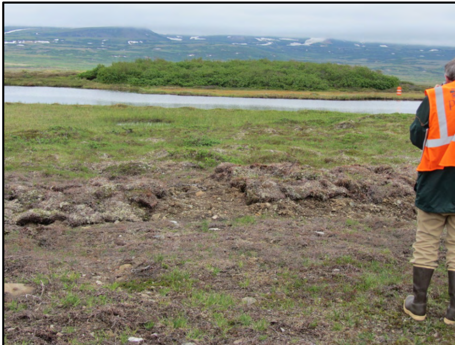
Photo #13. Sumps mounded as subsidence will occur during reclamation.
