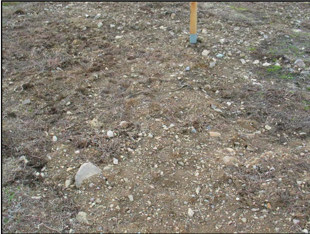
Photo #16. Disturbed area where hydraulic fluid was spilled. Contaminated soil and vegetation were removed and disposed of.
