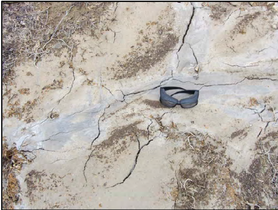
Photo #9. Desiccation cracks in remnants of discharged materials from previous artesian upwelling. No active upwelling has been detected since grouting. The site has not been remediated. Monitoring is ongoing to evaluate the efficacy of recent grouting efforts.
