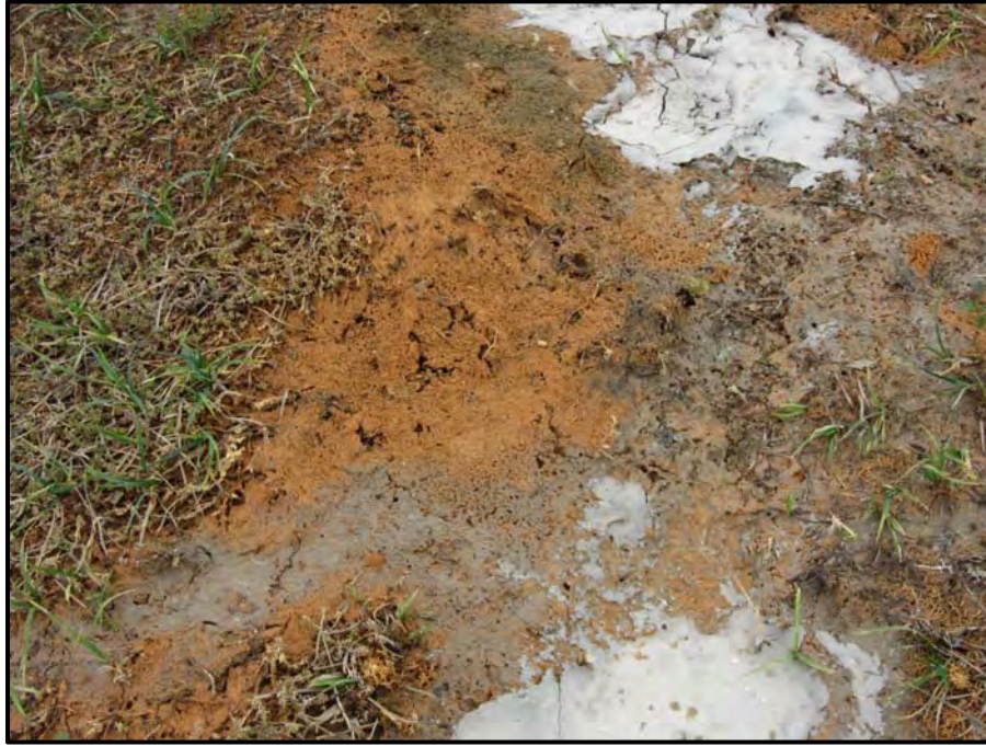
Photo #8. Staining from previous artesian upwelling
