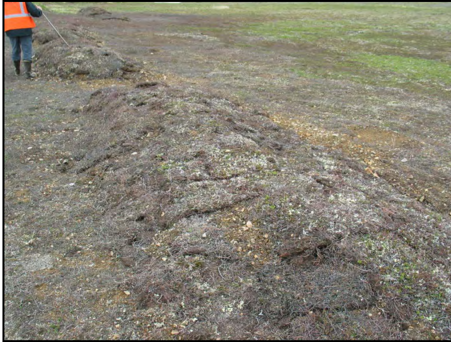
Photo #11. Pits filled and tundra replaced.
