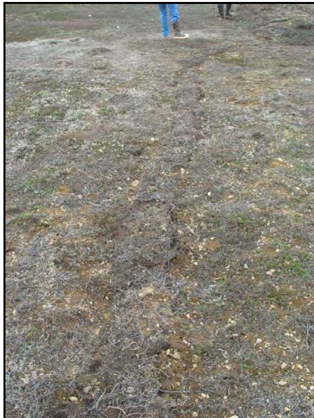
Photo #12. Fill and replaced tundra on discharge trench.
