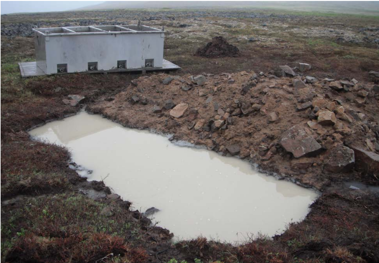
Figure 8 – DH 11532 Sump Pit and Recirculation Tank
