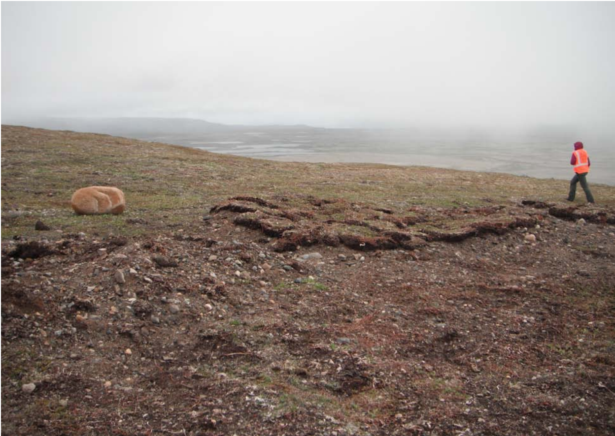
Figure 14 – DH 10514 Reclamation – Sump Pits – Site still settling
