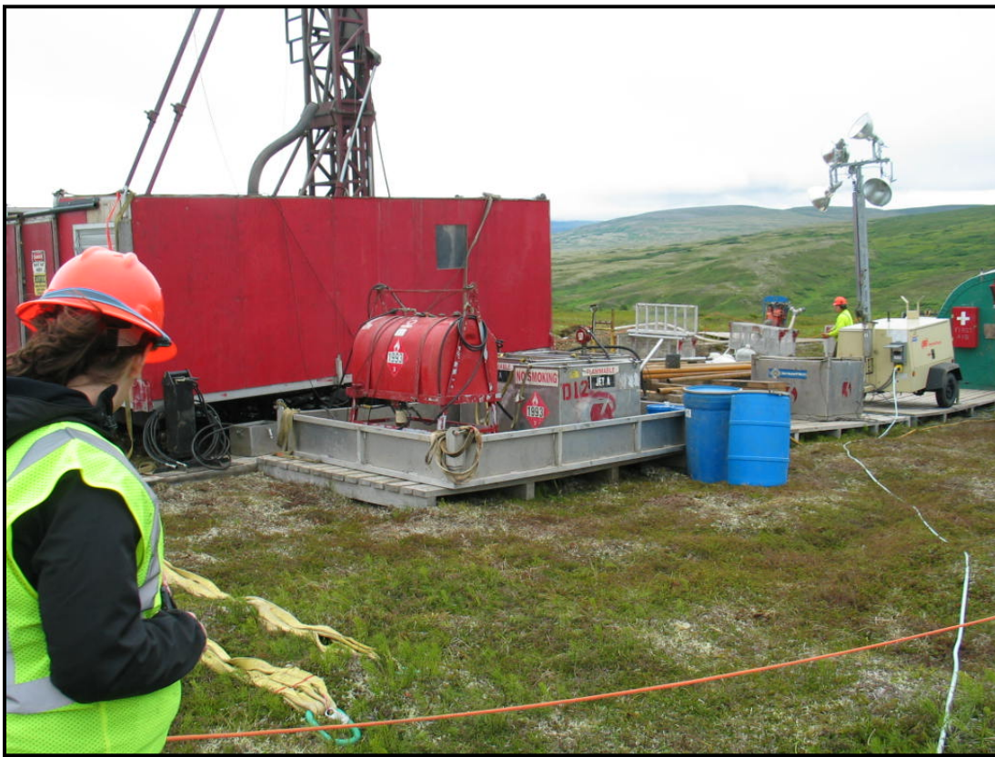
Figure #3. Drill #3. Fuel containment, spill kit, and scrubber barrel.
