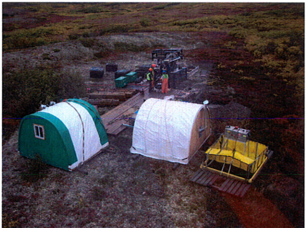
Figure 6. Drill rig 9, geotechnical drill hole.
