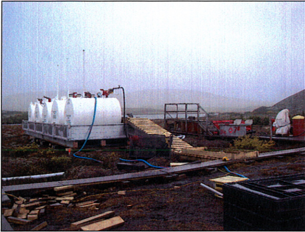
Figure 1. Fuel storage facility, former site on right side of picture.
