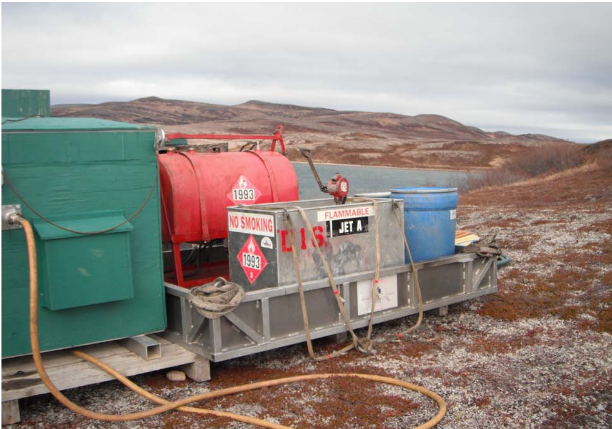
Drill Rig #3 – Drill Hole 10523 - Fuel Containment and Spill Kit
