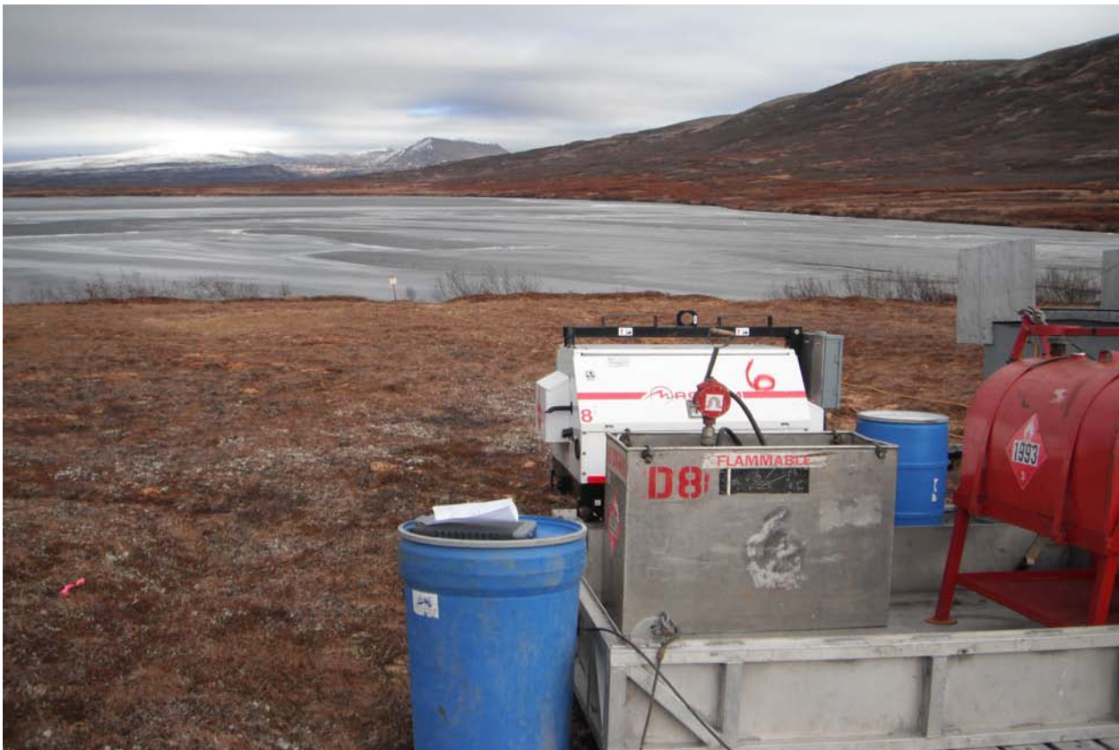
Drill Rig #2 – GH 10266 – Water Source Pump Location and Fuel Containment
