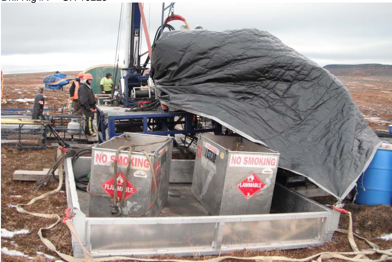
Drill Rig #1 – GH 10225 – Fuel Containment and Spill Kit
