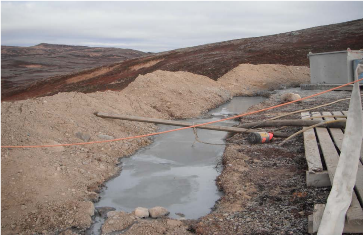
Drill Rig #3 – Drill Hole 10523 – Sump Pit
