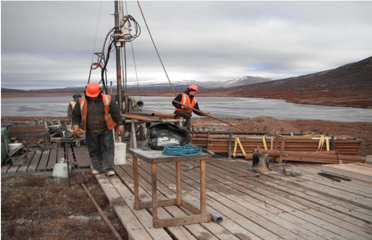
Drill Rig #2 – GH 10266 – Frying Pan Lake in Background
