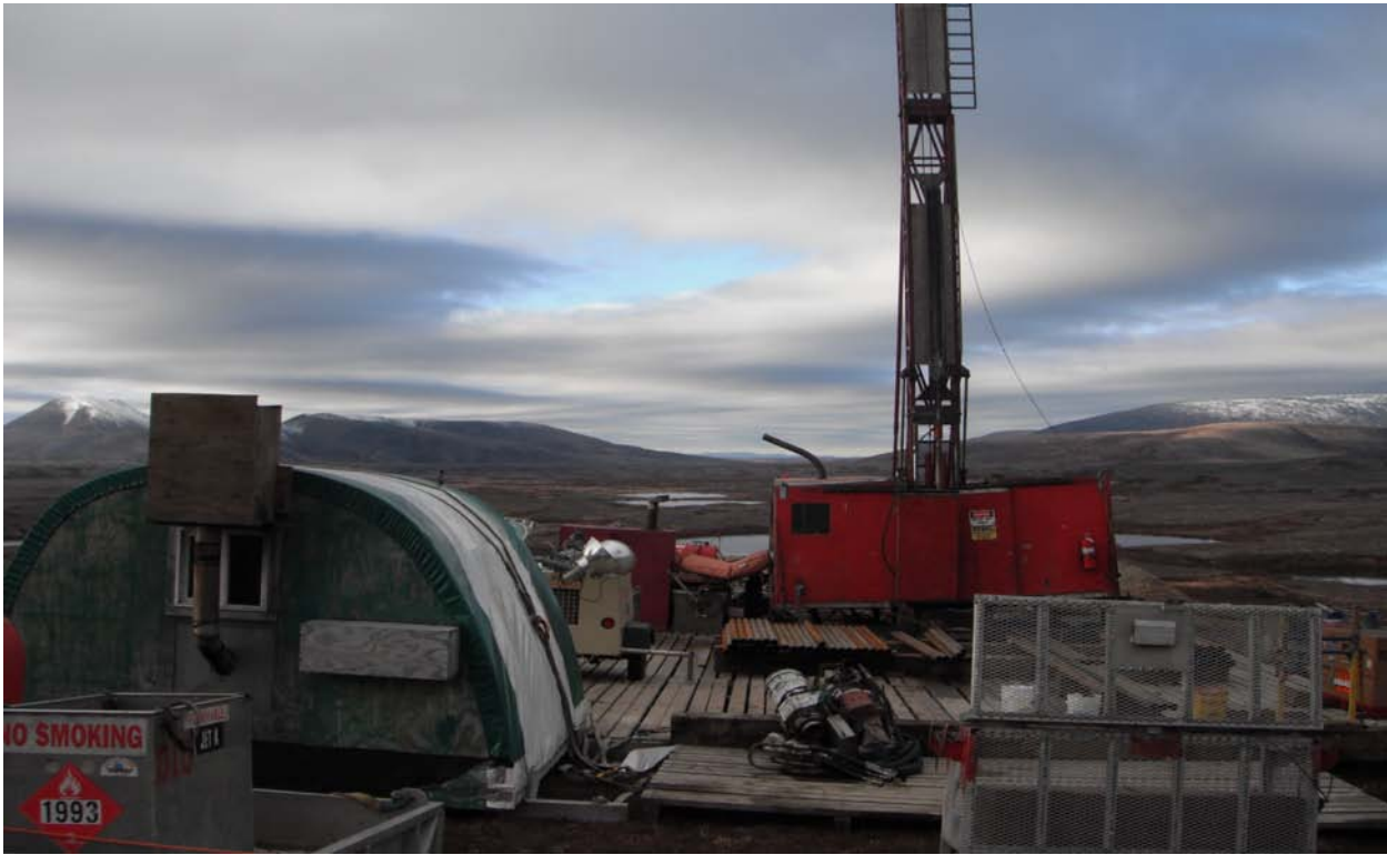
Drill Rig #3 – Drill Hole 10523
