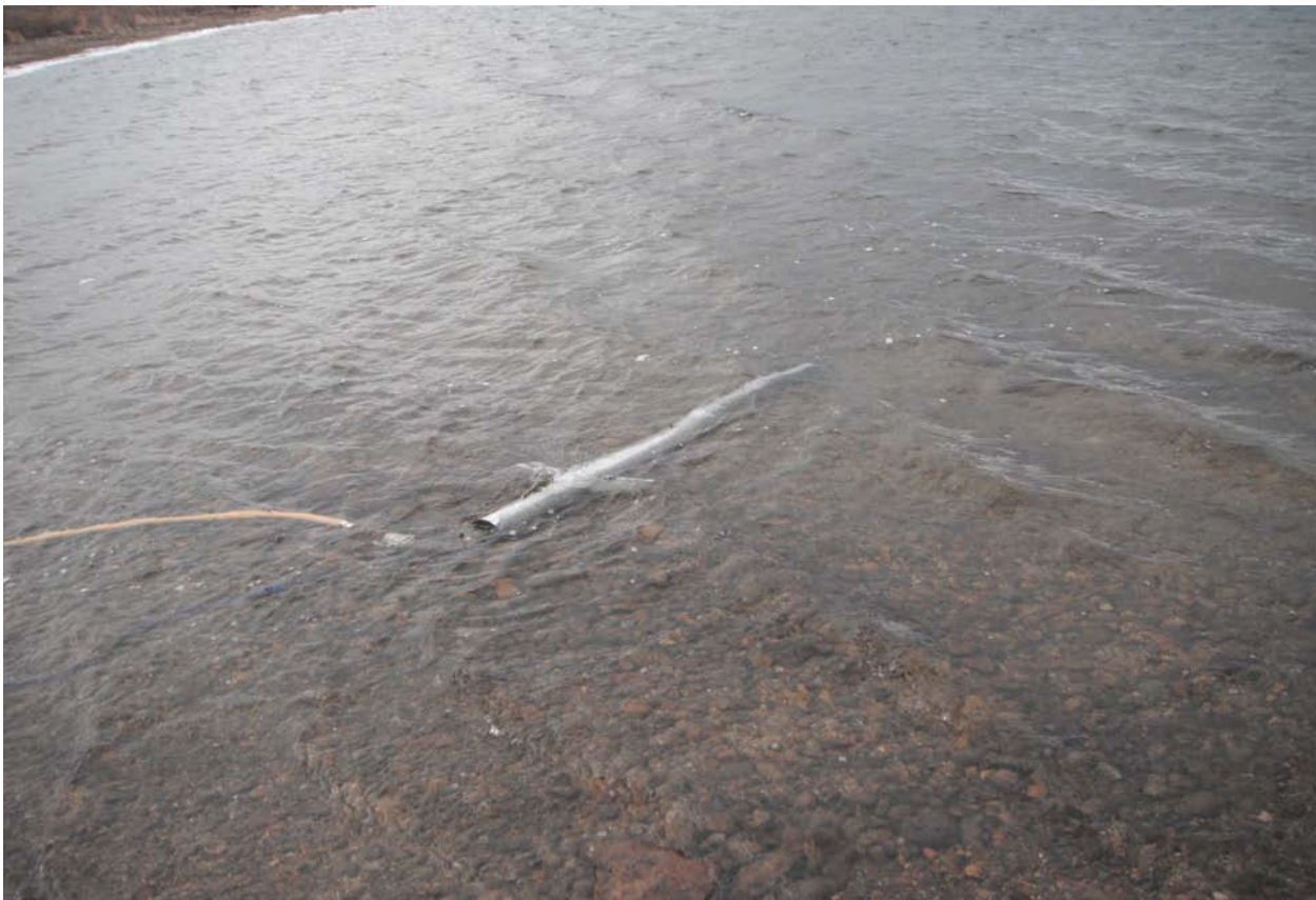
Drill Rig #3 – Drill Hole 10523 – Screened Intake Structure
