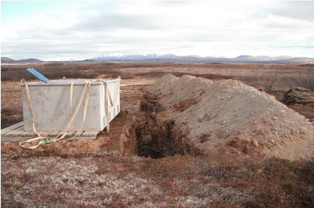
Drill Rig #4 – DH 10524 – Sump Pit and Water Recirculation Tank
