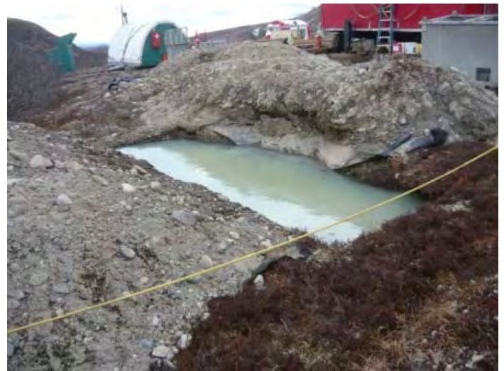
Lower sump pit and excavated material, DDHH 11541.
