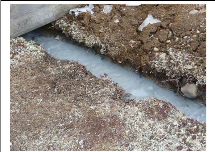
Recirculation flowing in keyway trench from drill rig.
