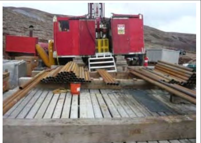
Drill rig #2, pipe stacked on tundra pad, DDHH 11541.
