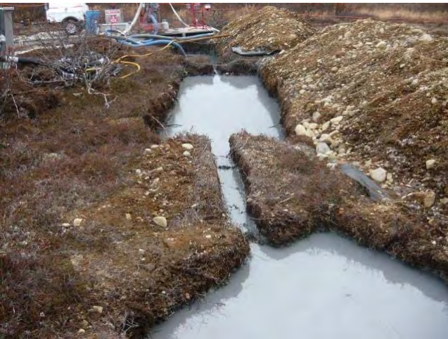
Sump trench #3 outlet to trench #4, soil stockpiles.
