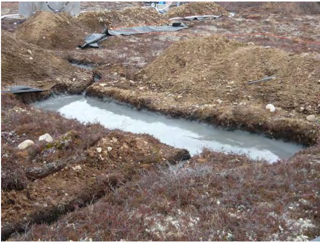
Keyway inlet into first sump pit, rig #6, site 11540.
