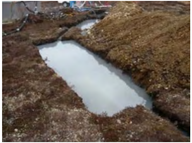
Sump trench #3, (4 in background), soil stockpiles.
