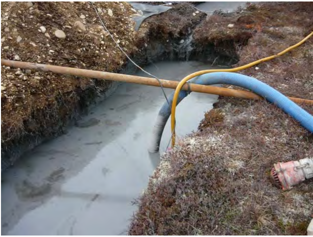
Blue suction hose to Godwin pump, sump trench #5.
