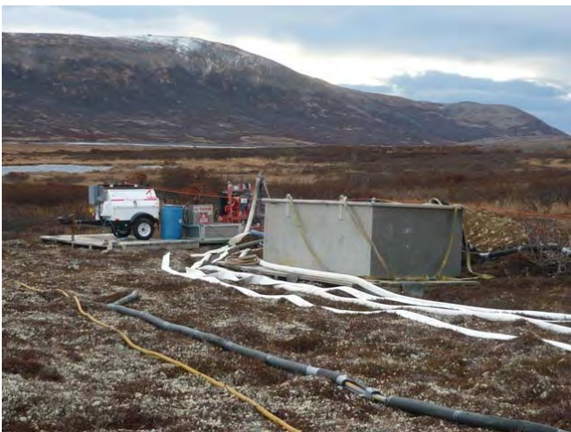
White outfall hoses running uphill from Godwin pump.
