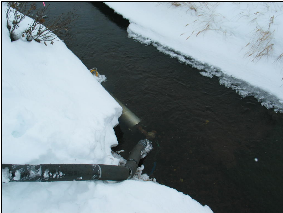
Photo #32. Water intake for drill #6.
