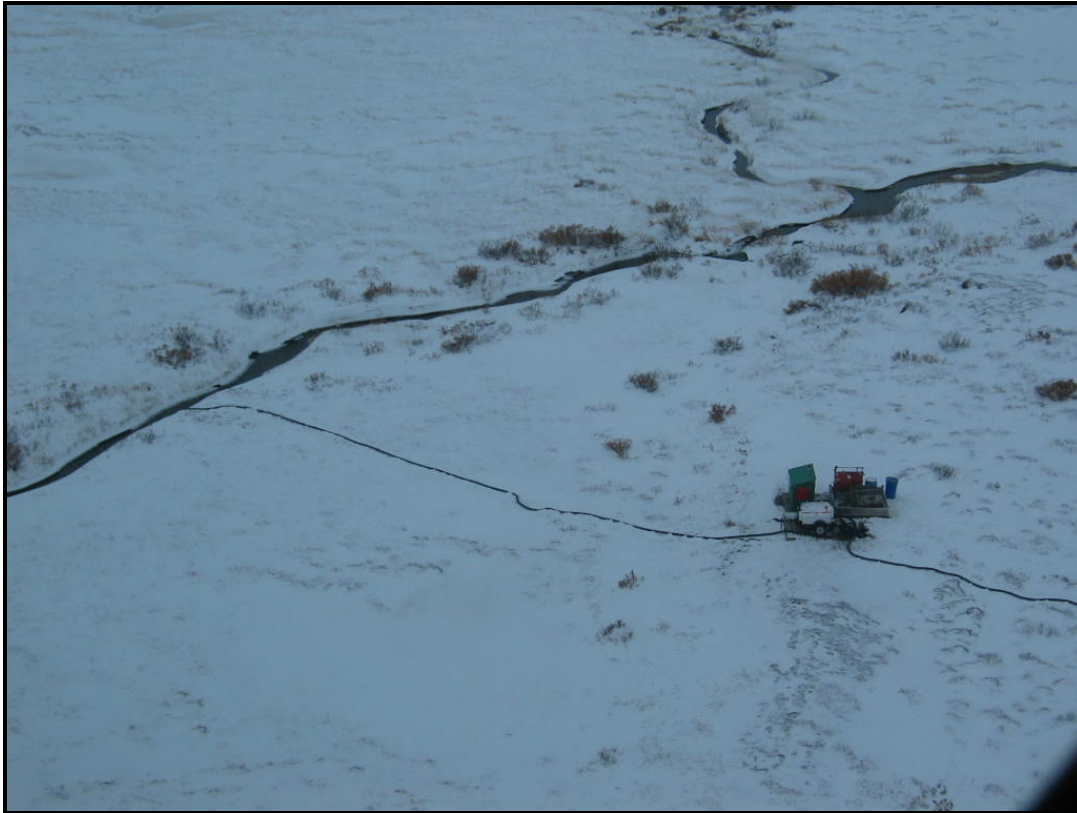
Photo #31. Water pump and intake stream for drill #6.
