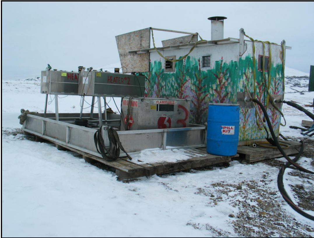
Photo #17. Shed and fuel containment at water pump for drill #3.
