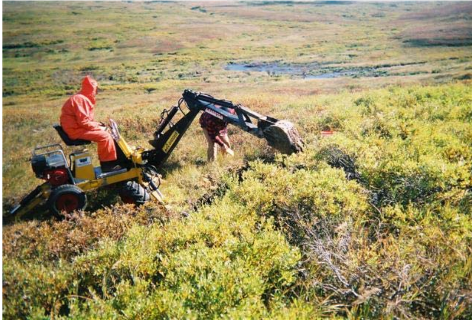
FIGURE 14-15: Another geotechnical test pit monitored by Amy Tomson. The excavators had an advantage in that they could dig much deeper than hand shoveling in the difficult glacial rubble.
