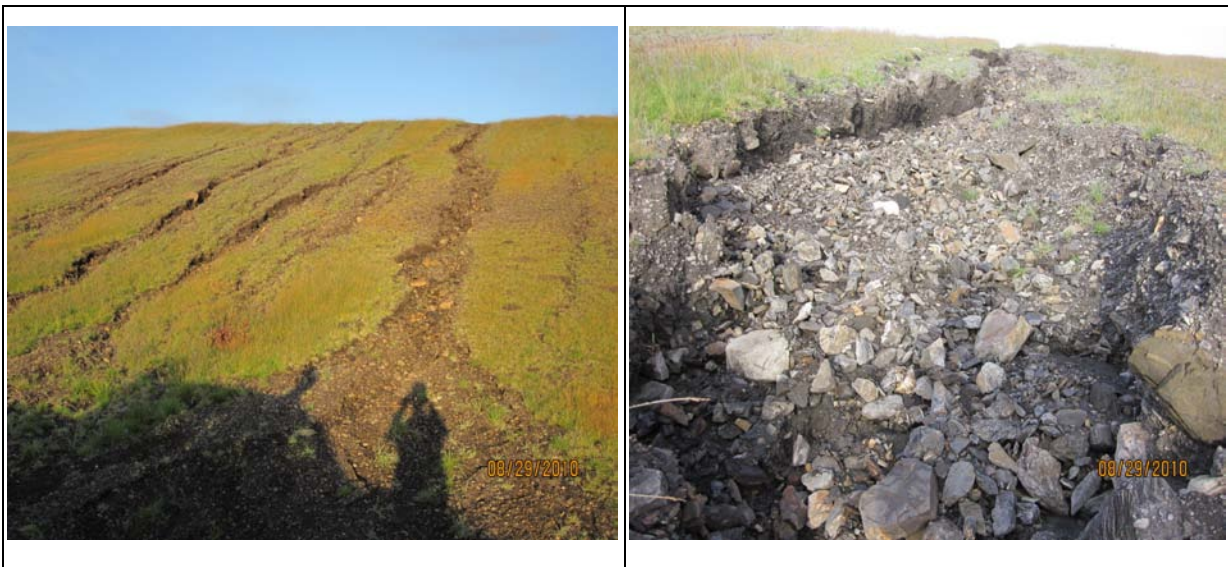
Figure 2.1 Areas of concentrated erosion rills on eastern slope of Oxide stockpile.
