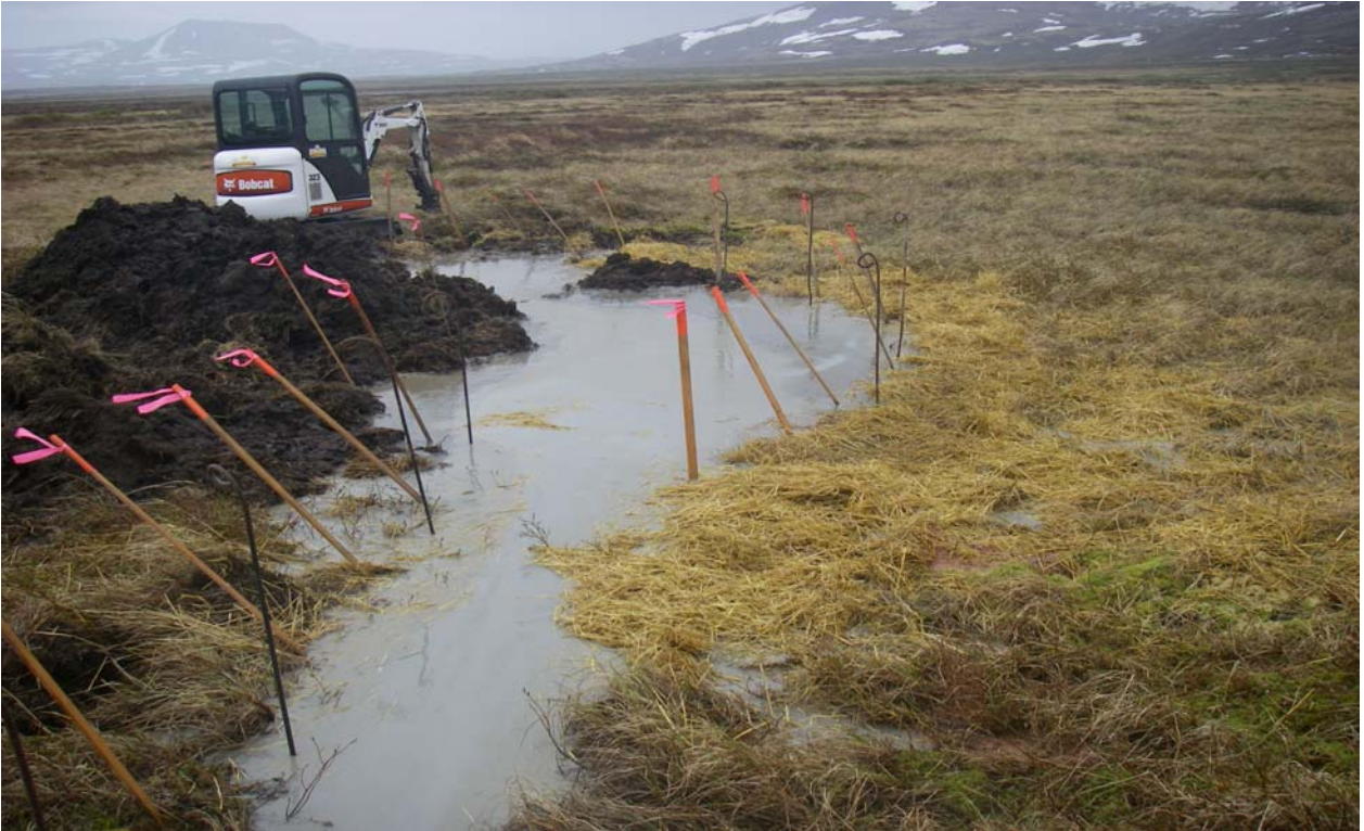
Sump Pit- Site #9451
