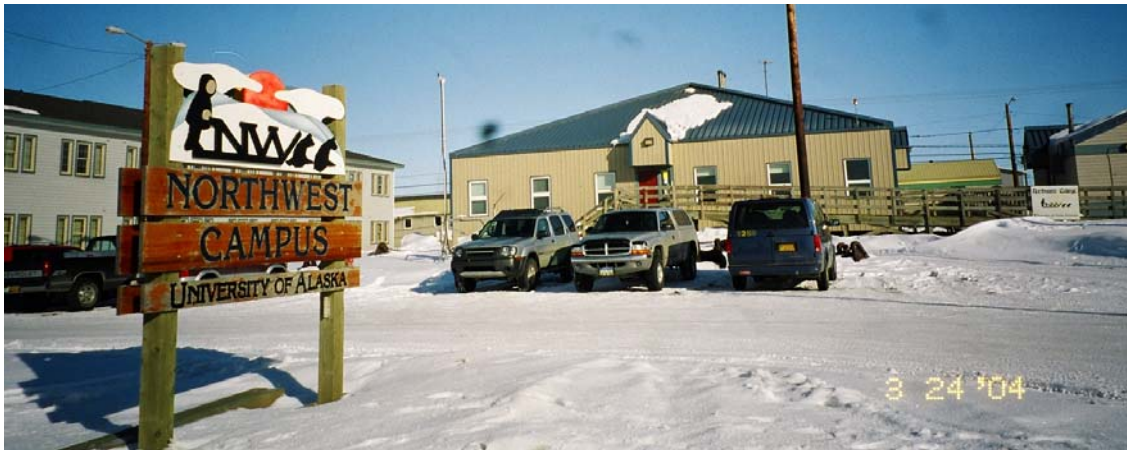
Figure 3-8: Northwest Campus, University of Alaska, Nome, Alaska.
