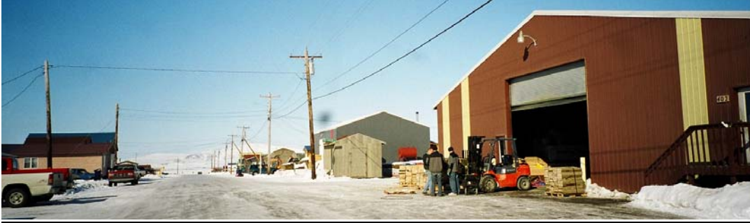
Figure 7-3: Industrial Buildings and Activity within Icy View residential subdivision, Nome
