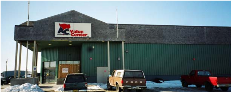
Figure 2-6: AC Value Center in Nome, Alaska
