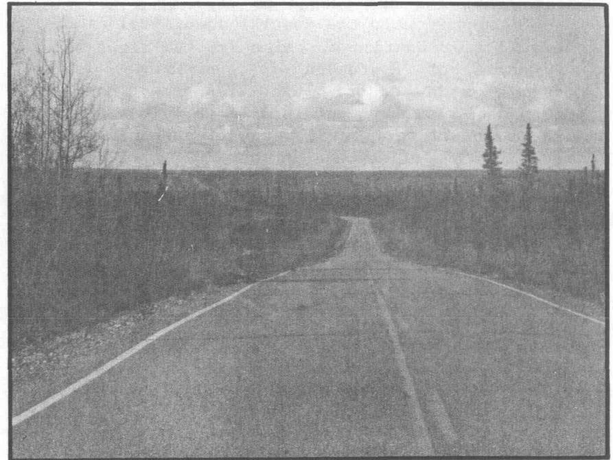
*Proposed road realignments would straighten curves on portions of the central Richardson. However in this relatively flat terrain, long, straight road tangents also increase visual monotony.*
