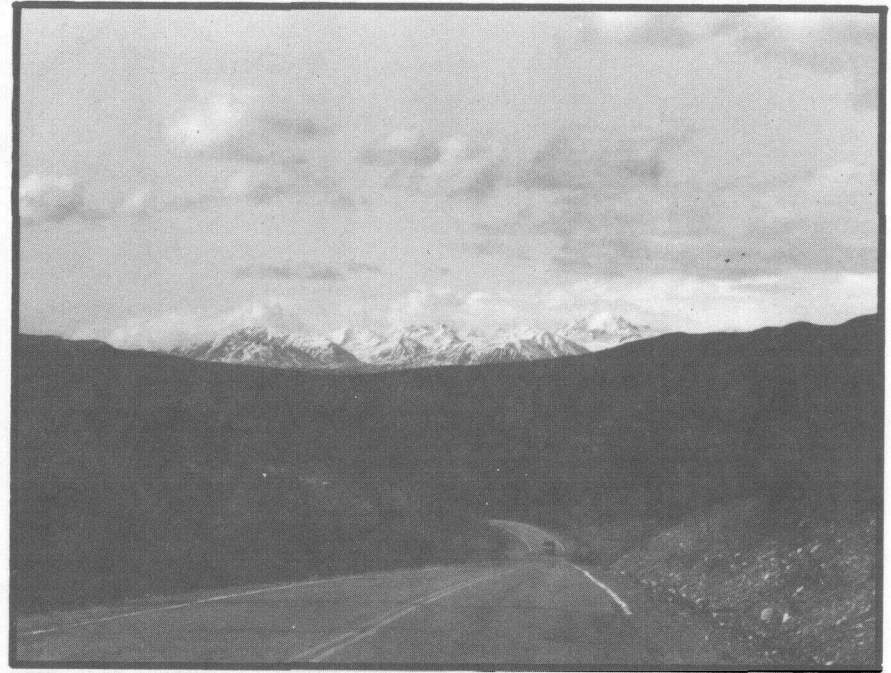
A relatively straight alignment, paved bed and graded shoulders allow faster, high volume travel and give this section of the Richardson its "highway" character.
