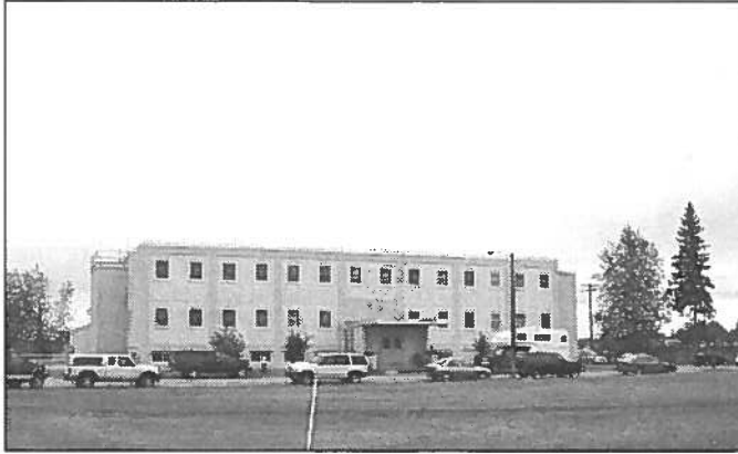
Figure 13. Site of Arctic Aeromedical Lab. Summer 2000.
