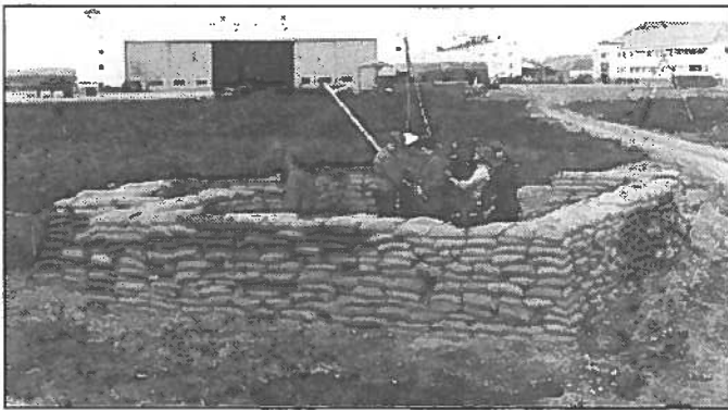
Figure 8. Ladd AAA emplacement. USAF photo 33257, Eielson History Office.
