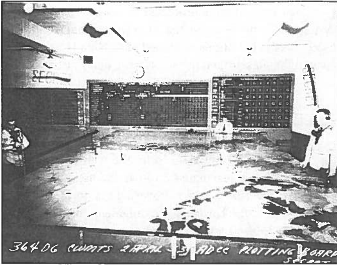
Figure 7. Interior of Air Defense Command Center, 1953.
