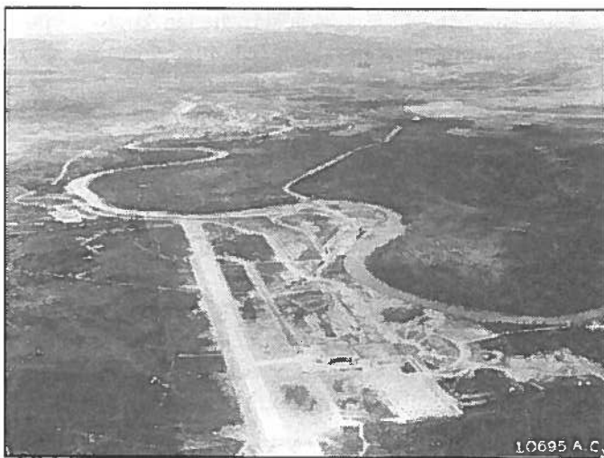
Figure 15. Ladd Runway, ca. 1943. USAF photo 10695, Eielson History Office.
