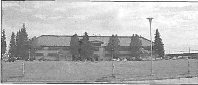
Figure 9. Headquarters, Bldg 1555. Summer 2000.
