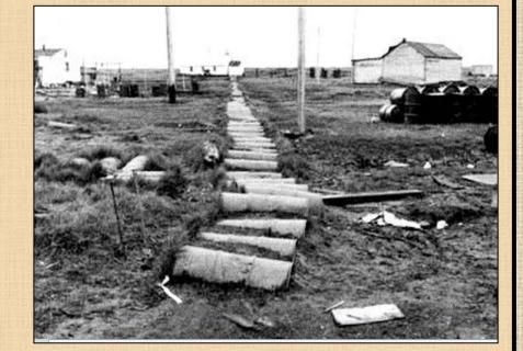
Figure 21. A tundra walkway through a village consisting of a linear series of drums
