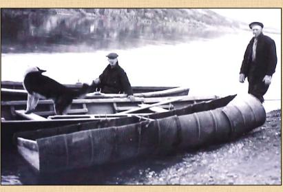
Figure 16. Four drums welded together to form a canoe (1940s) (archival photo).
