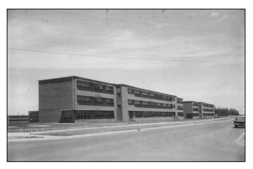
Top: This Korean-era barracks was built of concrete and steel and was known as the "Hammerhead" barracks, because in plan and from the air, it resembles a hammer.
