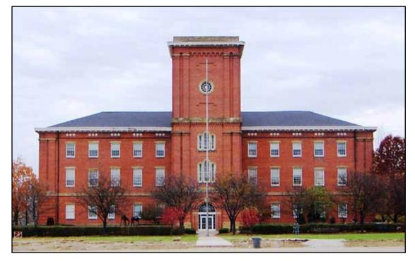
Top: The Storehouse (1863) at Fort Hayes, Ohio (originally Columbus Arsenal), is dominated by the central tower. Other defining features include the symmetry, hip roof, cornice, and use of round arches in the windows and entrance.
