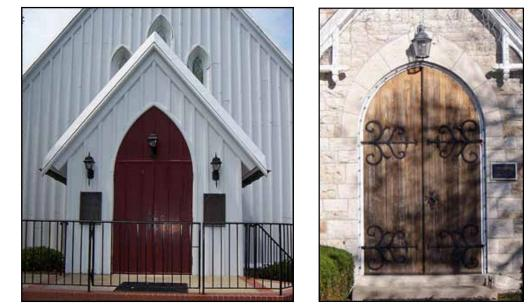
Both of these doors have pointed arch forms and vertical board construction. The one on the right also has the decorative iron strap hinges.
