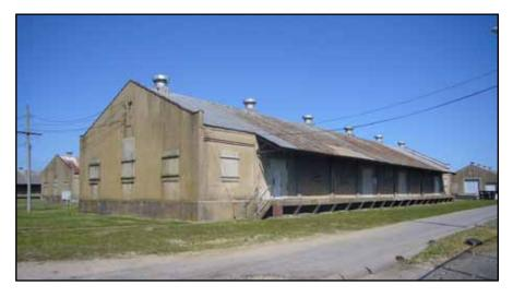
Gabled ends, covered loading docks, horizontal massing, and roof ventilators are characteristic of storage and warehouse buildings, as shown at this concrete storehouse building (ca. 1918) at St. Julien's Creek Annex (NSA Norfolk Naval Shipyard), Virginia.
