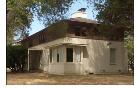
Top: The Thermo-Con House (1948) at Fort Belvoir, Virginia, was designed by Albert Kahn and uses the experimental Thermo-Con material, which expanded as it cured. The house is designed in the International Style, exhibited by the flat roof with overhanging eaves, smooth wall surface, and cantilevered canopies.
