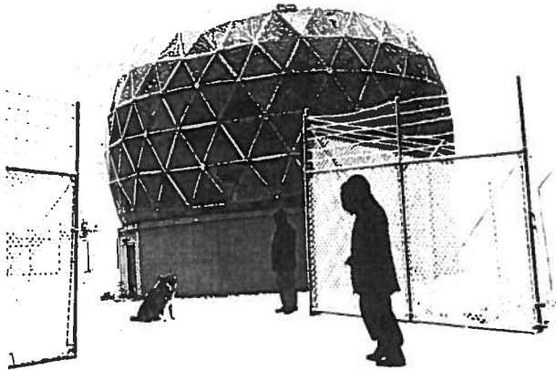
Figure 8.3 Pacific General Construction Company workmen are shown closing in the dome of a High-Power radar facility at Site Summit Nike Station near Anchorage.
