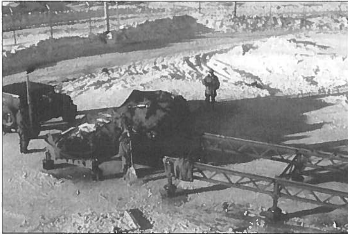
Figure 7: Site Summit launch building before installation of rails and launcher. Courtesy Bill Momsen.
