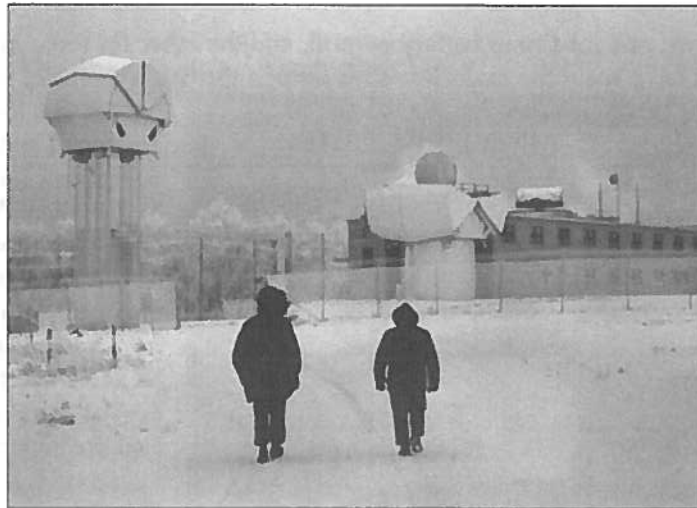
Figure 17: Missilemen walking to Control Area of a Fairbanks Nike site, 1962. Note open clamshell cover on radar, right. U.S. Army Photo.
