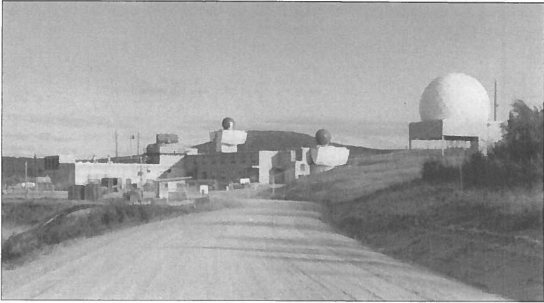
Figure 12: B Battery IFC area, 1970, Fairbanks. Courtesy Jim O'Connor.
