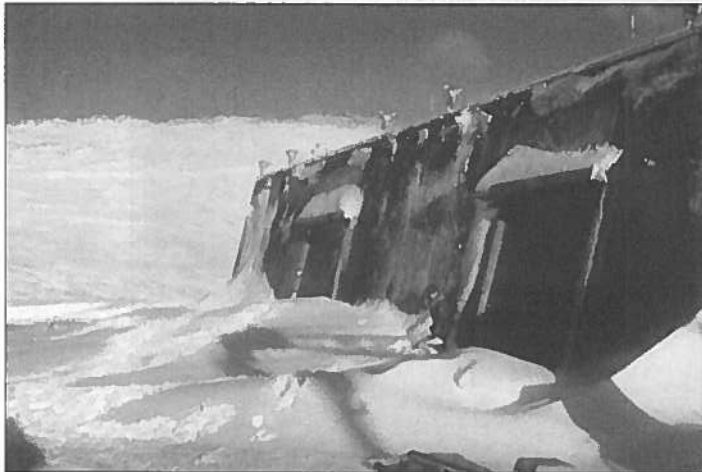
Figure 8: Site Summit, installation of launcher and rails. Note crewman with broom - an essential tool, according to Billy Momsen. Courtesy Bill Momsen.
